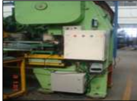
Instillation of VFD's
