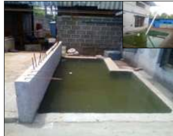
Rain Water Harvesting Tank (capacity 10 kl) Near Compressor Room
