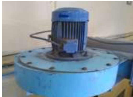
Powder Recovery Blower Motor (2 HP )
